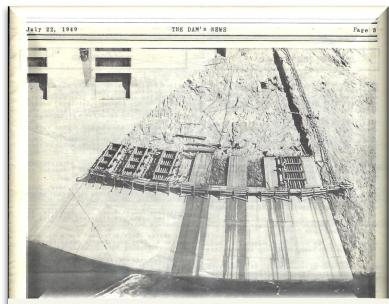
PLACING CONCRETE SLOPE PAVING ON RADIUS CORNER UPSTREAM FROM INTAKE STRUCTURE
